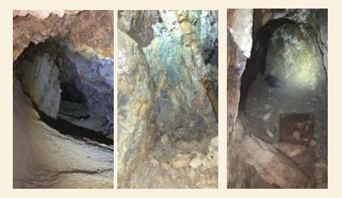
Historic artisanal workings have left a well-preserved network of underground drives at Aurora, providing immediate access for detailed mapping and systematic sampling.
